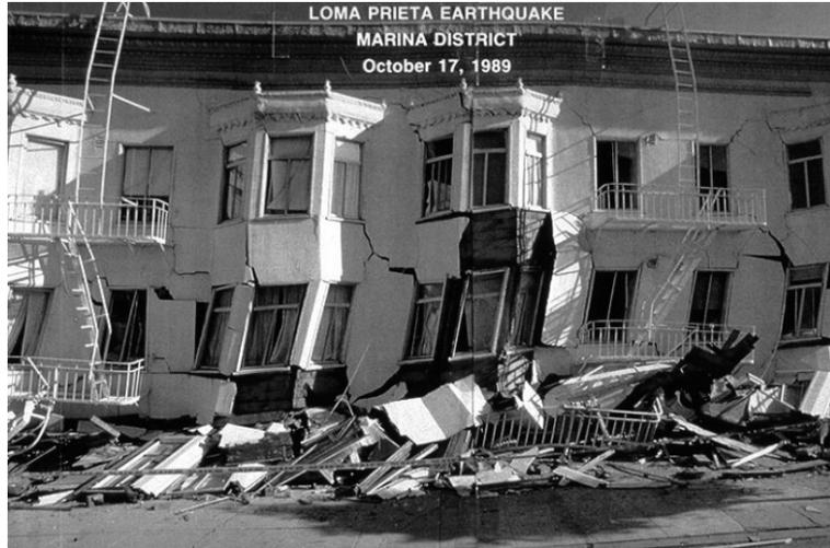
**Figure 2** Marina District Apartment building damage during the 6.9 magnitude 1989 Loma Prieta earthquake. Two nearby public schools were not damaged and were used as emergency shelters.
